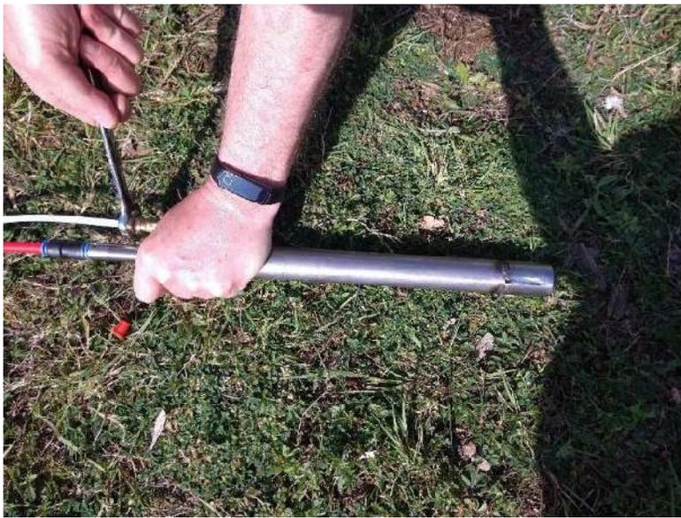
Using adhesive tape secure the hydraulic tubing to the anchor protective tube at regular intervals.
