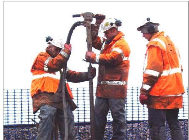
2. Once the barrels have been jacked out, lower the cone into the hole. It is crucial, at this stage to ensure that one set of internal 'grooves' is in line with the expected direction of movement.
