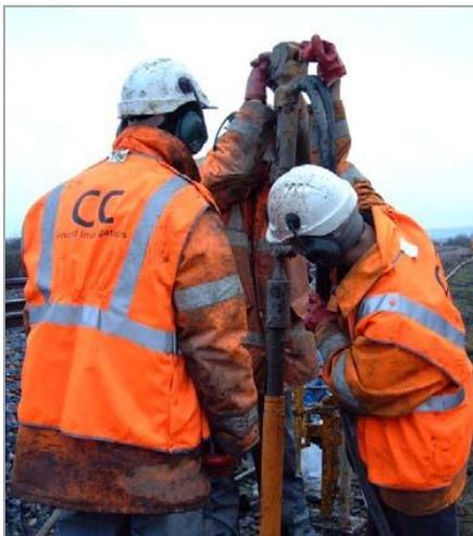
4. Pour a grout mix into the hole to act as a lubricant, reducing skin friction between the inclinometer tube and the sidewalls of the borehole.
